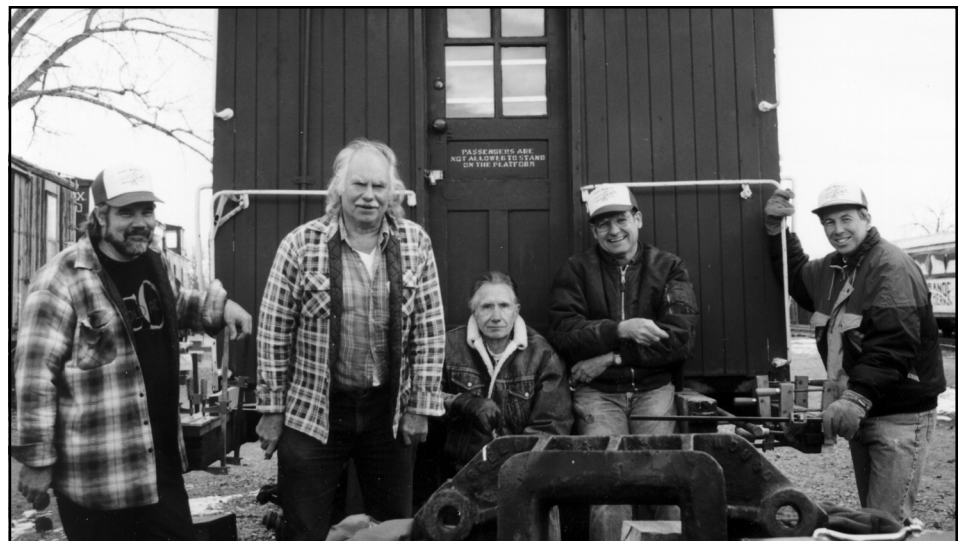
Working on caboose framing at the Colorado Railroad Museum were from left: Duane Fields, Bob Tully, Ralph Vance, Steve Mason and Ken Gow. – Photo © Steve Mason
